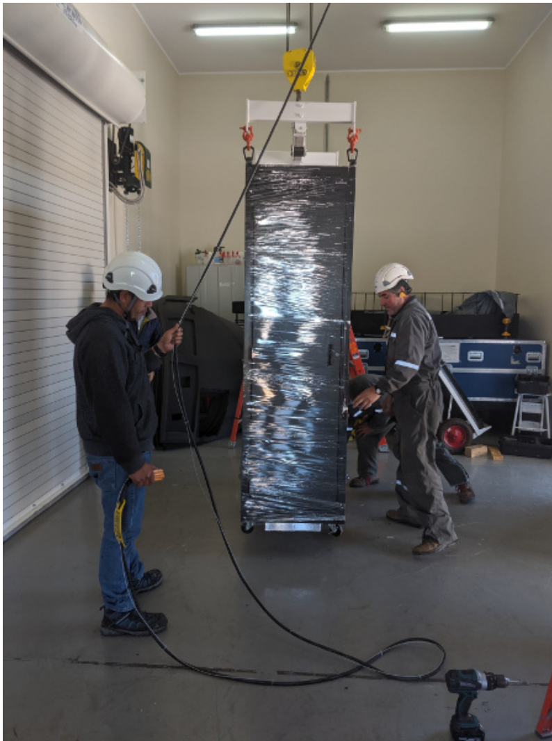
The electronics box rack being lifted.
